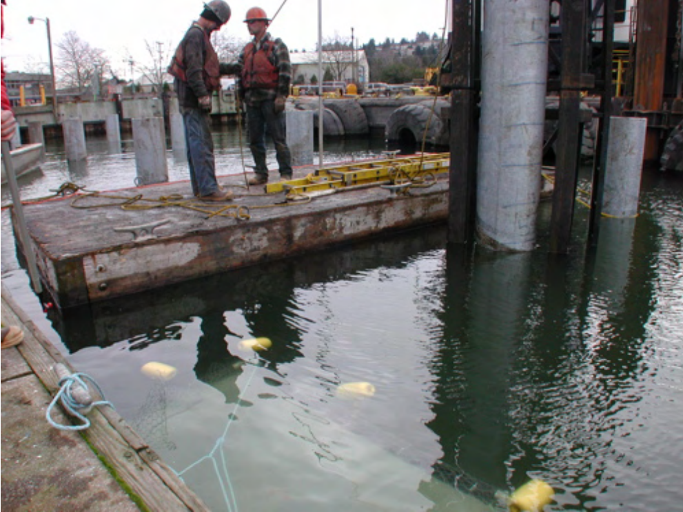
Salmon cage near pile to be hammered.
