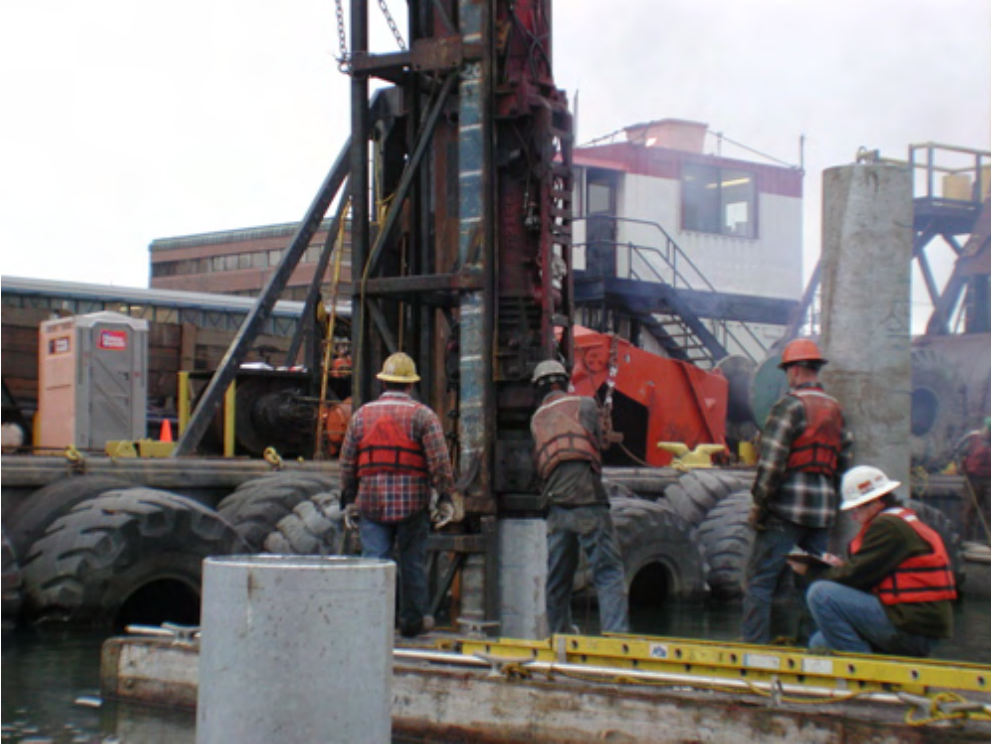
Impact hammer and crew. Steel pile in foreground.
