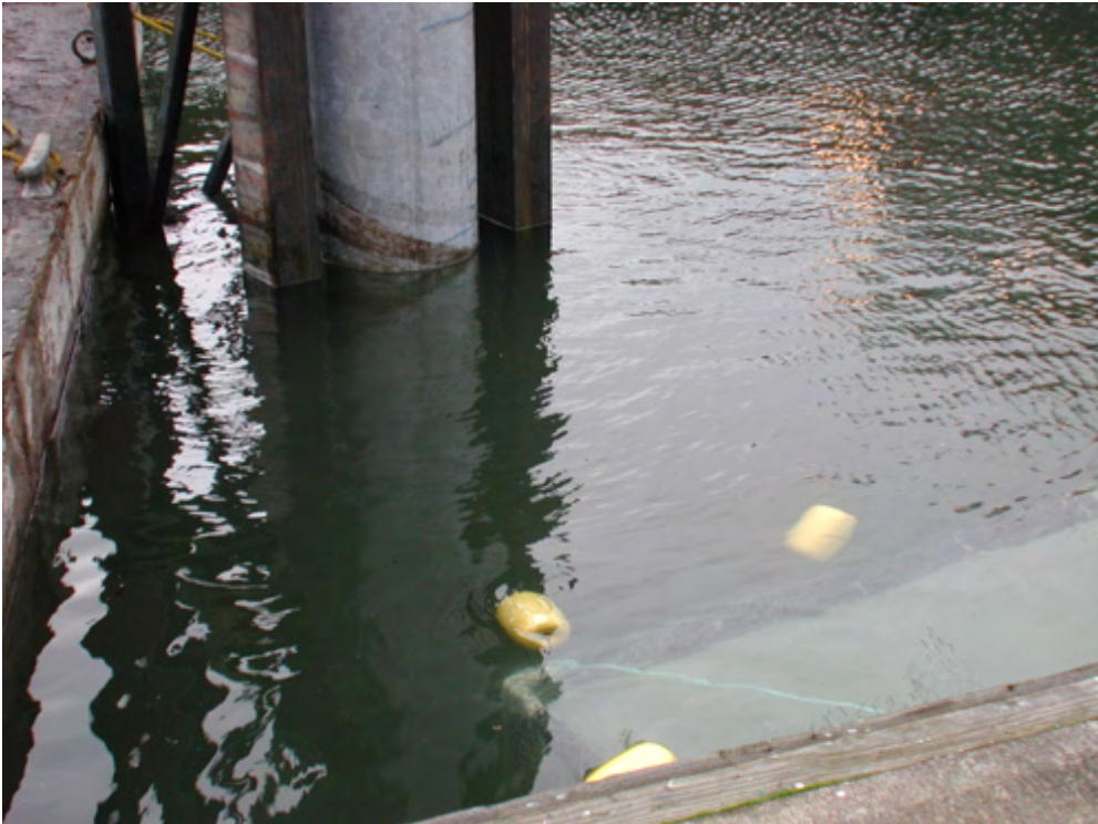
Salmon cage near pile to be hammered.
